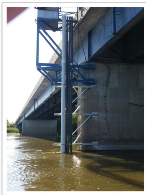
**Figure 16.2. - USGS Super Gage continuous monitoring station at Joslin on the Rock River (IEPA, 2021)**
